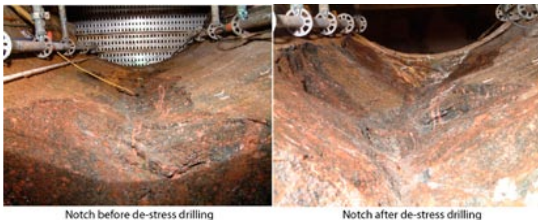
Figure 10-6. Photograph of the pillar taken in DQ0063G01 from a depth of approximately 3 m and up. The photograph on the left was taken before de-stressing began and the one on the right after removal of the slabs created during de-stressing.
