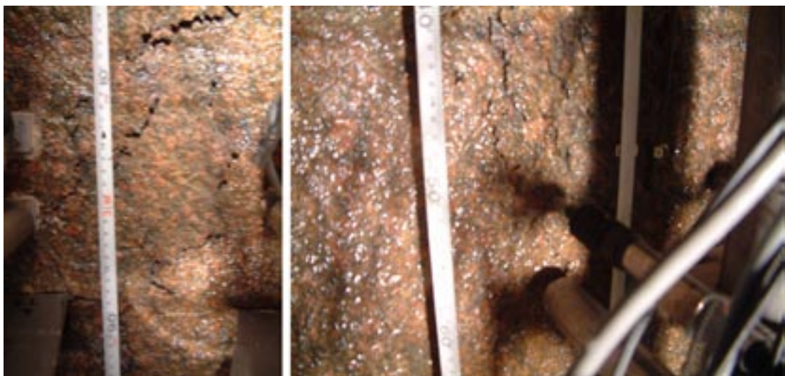
Figure A2e-20. June 29. Photographs of spalling/fracturing at position 9 at the 3 m level (left) and at position 15 at the 3.5 m level (right).
