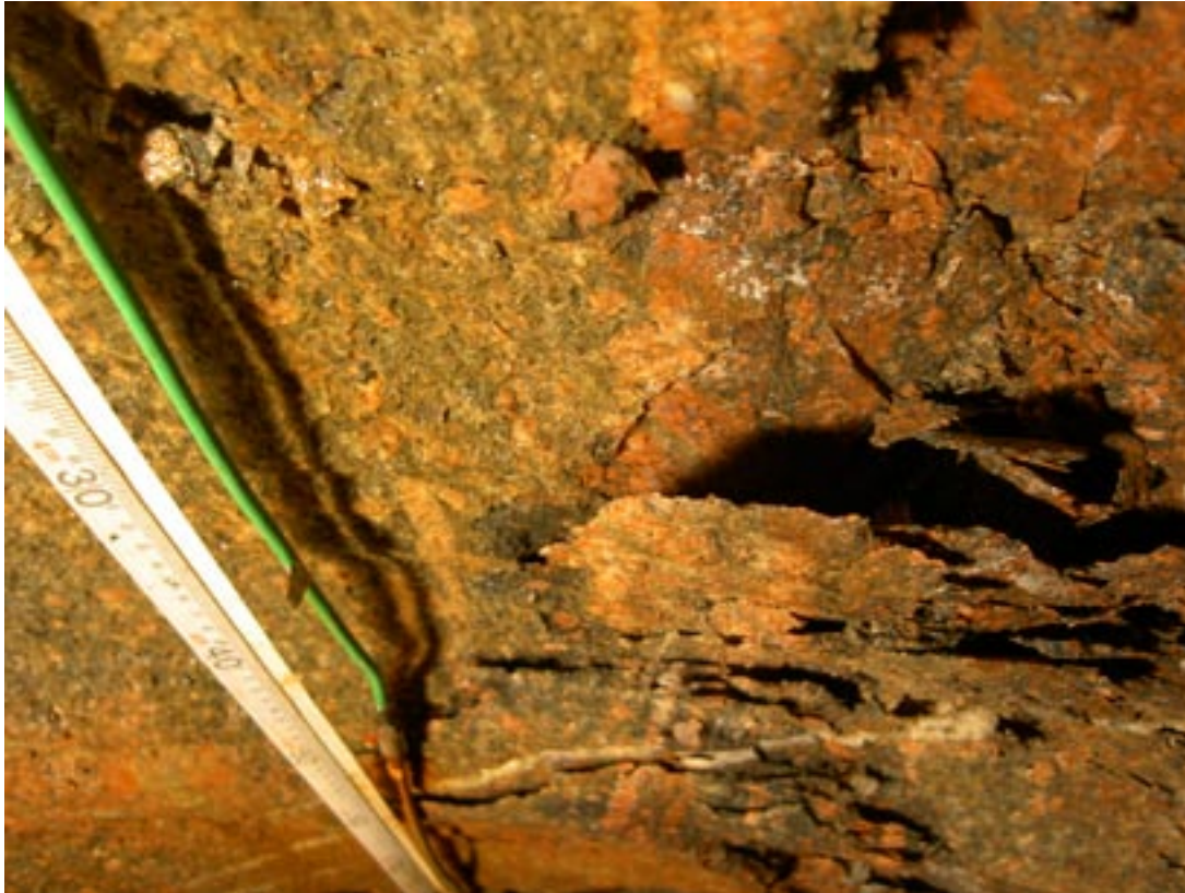
Figure A2e-26. Photograph of the upward-pointing chips.
