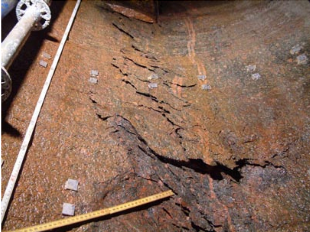
Figure A2e-30. Photograph of the slabs with a free left surface and the right side attached to the rock wall. The depth at the bottom of the photograph is 3 m.
