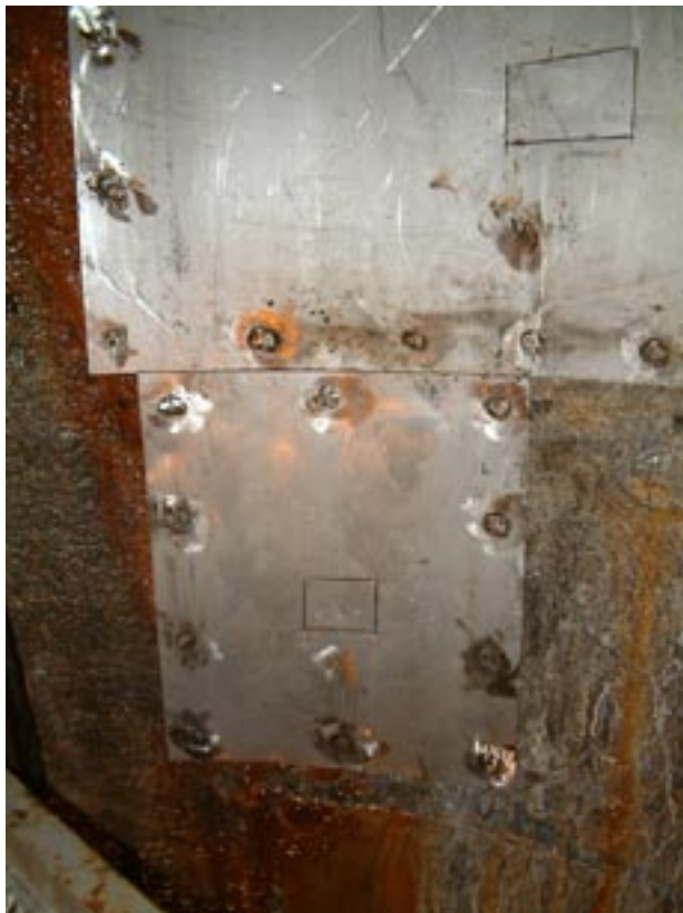
Figure 9-1. Photograph of steel plates bolted to the hole wall.
