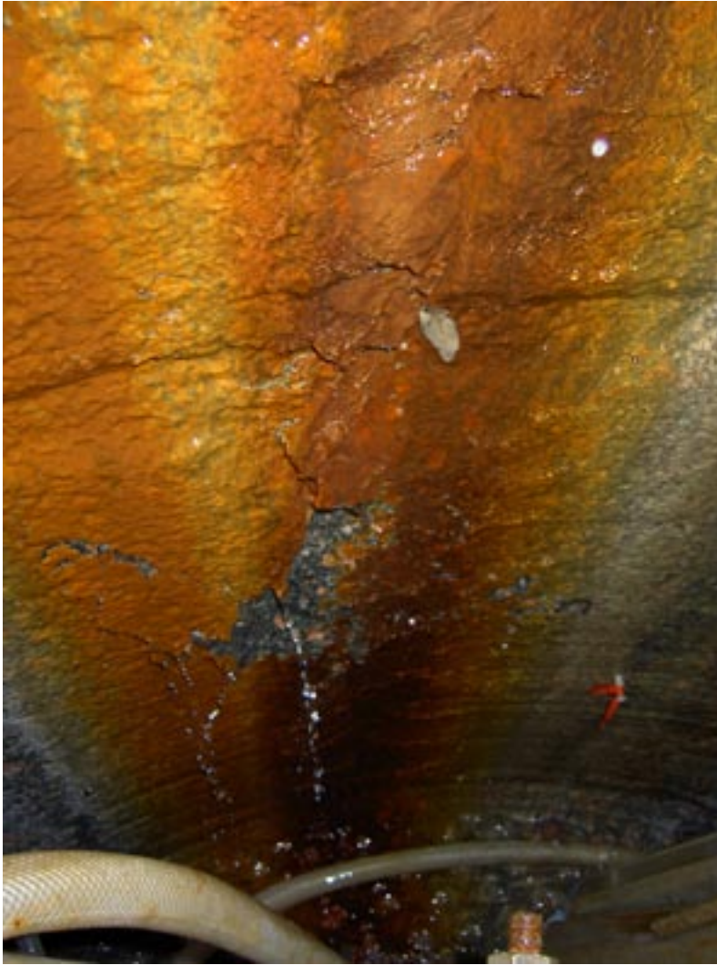
Figure 10-8. Yielding at the back side of DQ0063G01. Dilation of rock slabs and the previous location of the ejected rock piece are visible.
