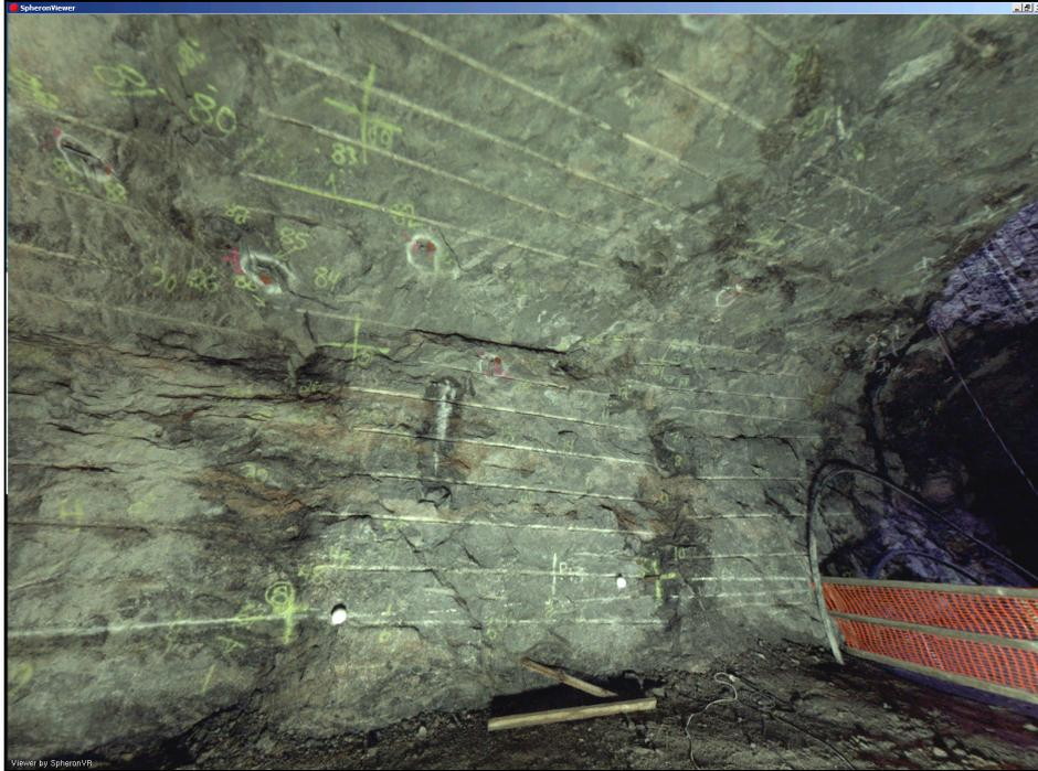
**Figure 16.** A laser scanning image in combination with high resolution digital photo. Scanning and photography took place simultaneously (Onkalo).
