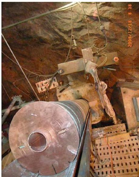
*Figure 4-5. Placement of clay blocks. Block column with copper plate fixed to the throughgoing central tube.*
