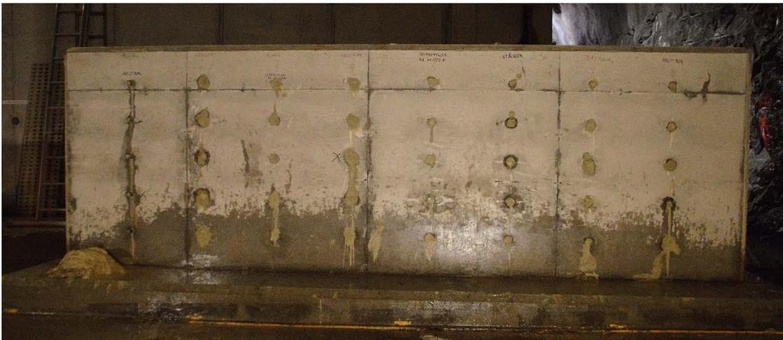
*Figure 3-10. The wall after that all tubes have been filled with grout.*
