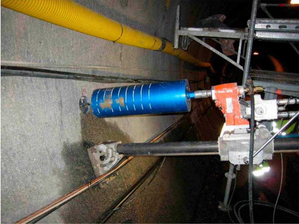
**Figure 3-3.** The LVDT-cell is installed inside the pilot hole just before overcoring in the Äspö hard rock laboratory TBM-tunnel (at about 450 m depth). The drill bit was marked every 50 mm for manual coring advance recording (Hakala et al. 2013).
