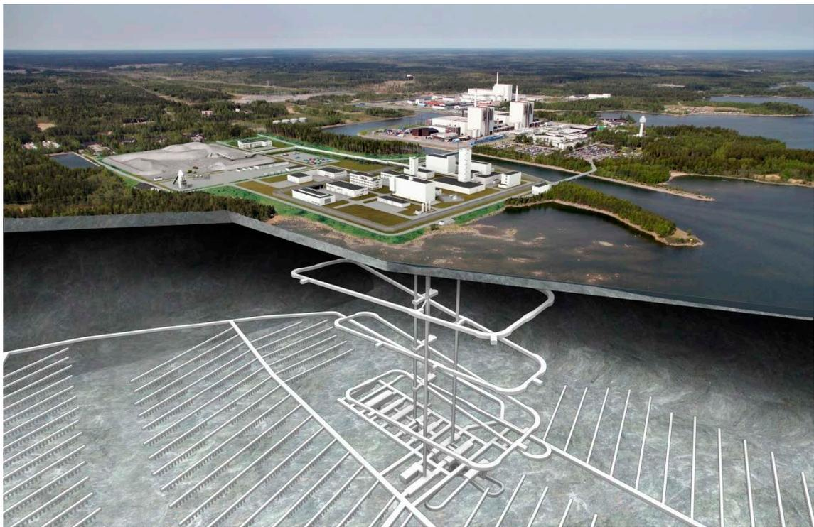
**Figure 1-4.** 3D-illustration of the planned facility for spent nuclear fuel.
