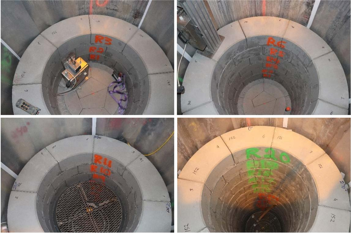
*Figure 4-5. Installation of ring layers. Top left: R3, Top right: R6, Down left: R11, Down right: R20.*
