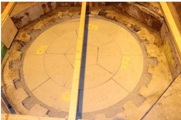
*Figure 4-9. The pellets are installed between the block and the rock.*
