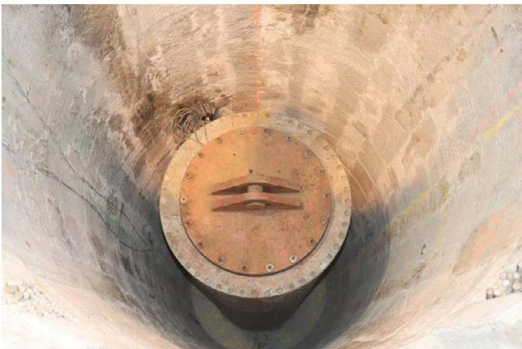
**Figure 5-14.** The canister is exposed in all its length and is ready to be lifted.
