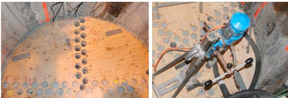
**Figure 4-16.** Left: Wood template used when core drilling. Right: Core drill.
