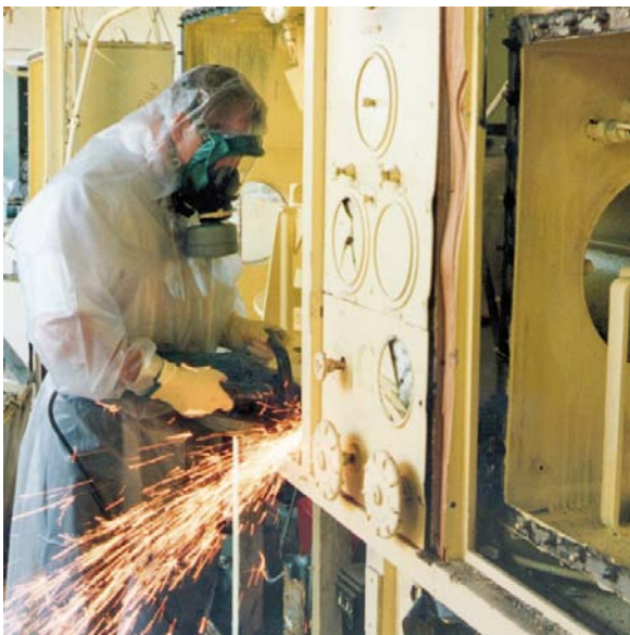
Figure 3-10. Typical manual plant dismantling operations.
