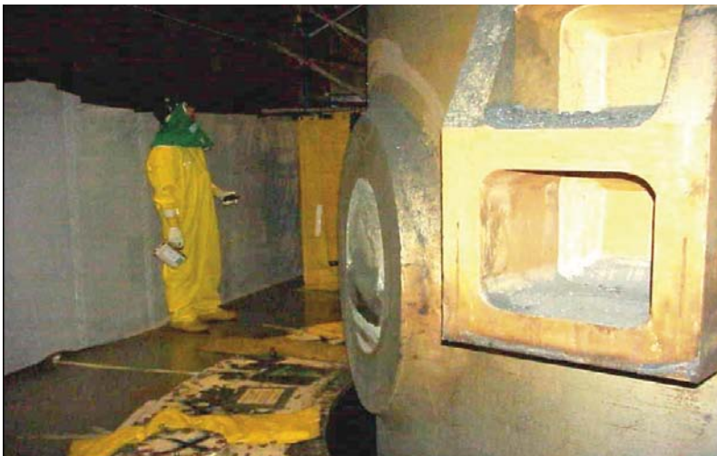
Figure A1-10. San onofre unit 1 reactor vessel nozzles after cutting with a diamond wire saw.
