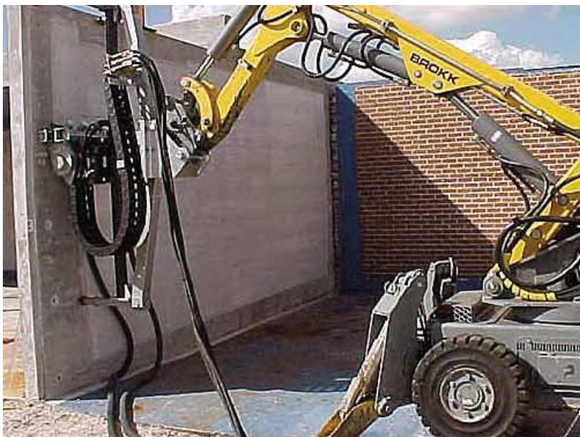
Figure A1-17. Shaver mounted on Brokk 250 for wall decontamination.
