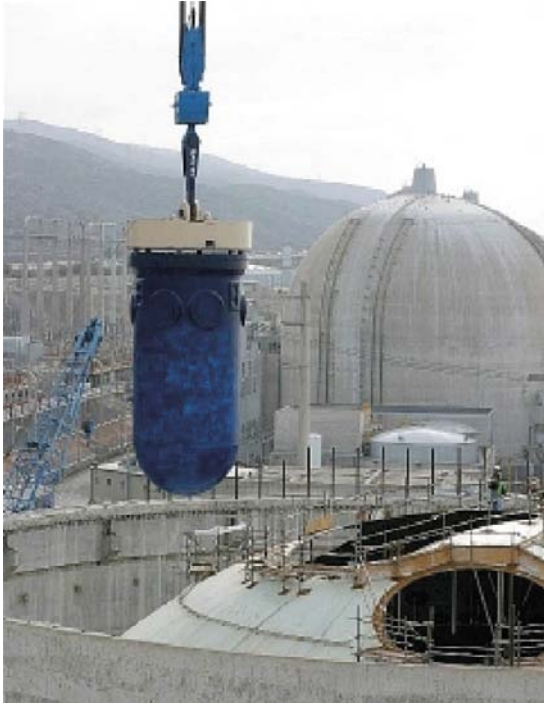
Figure A1-28. Removal of the San Onofre RPV via the reactor containment.
