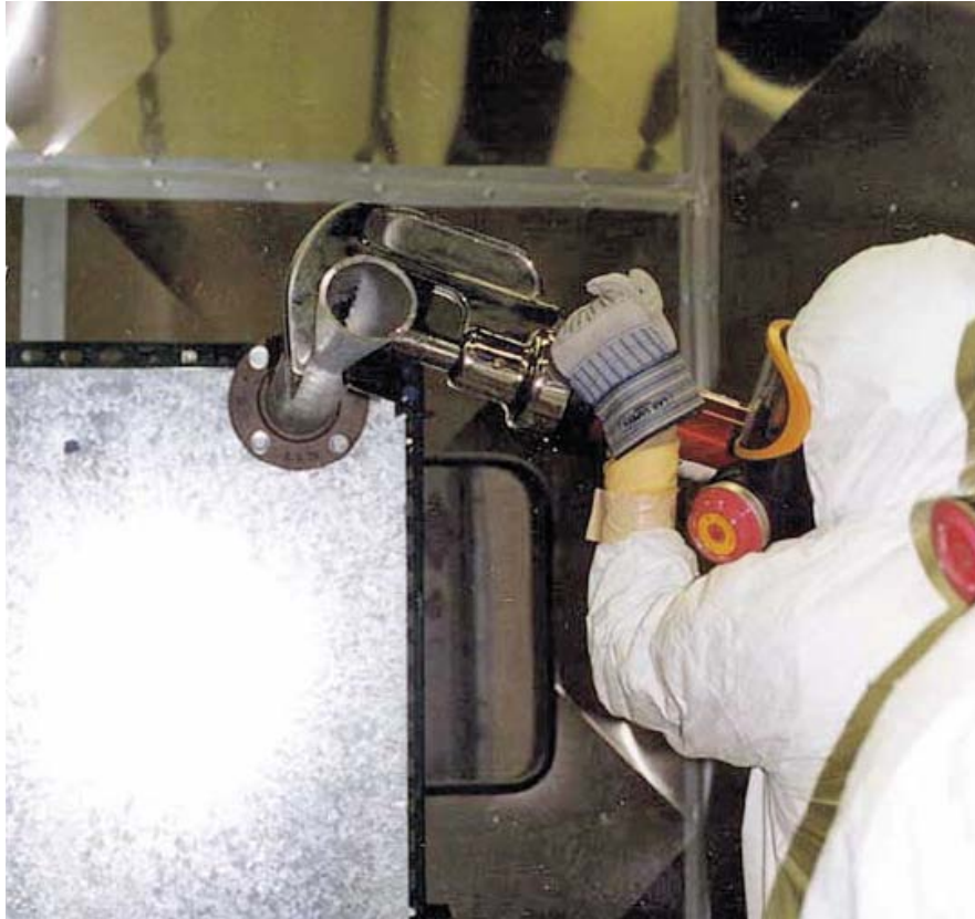
Figure A1-13. Mega Tech Blade Plunging Cutter being used to cut 2.5 inch OD pipe.
