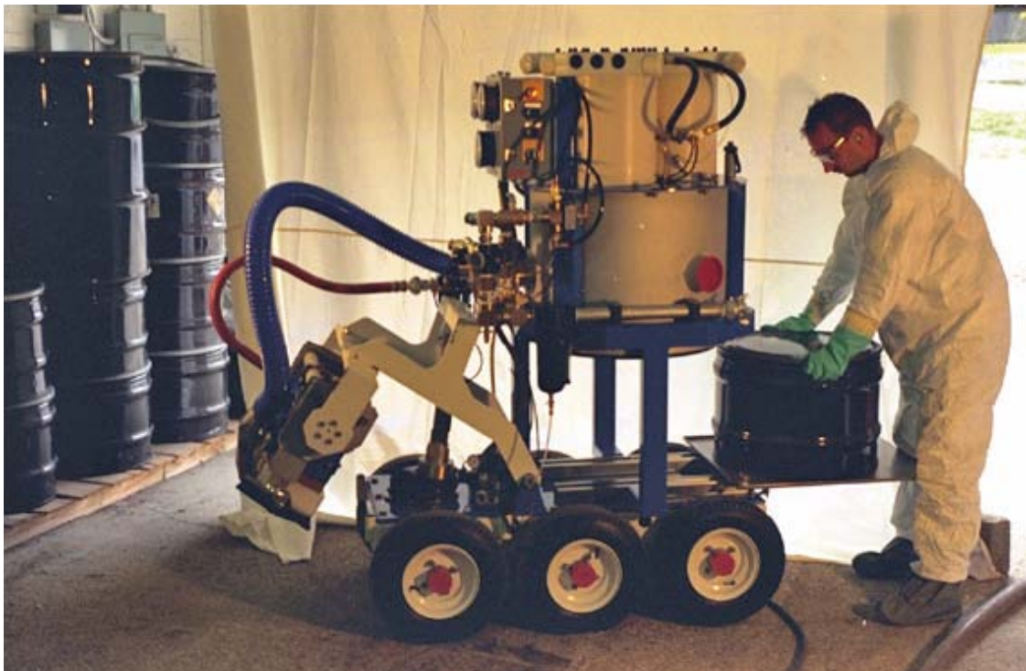
Figure A1-14. PENTEK Moose® Remotely Operated Floor Scabblers.
