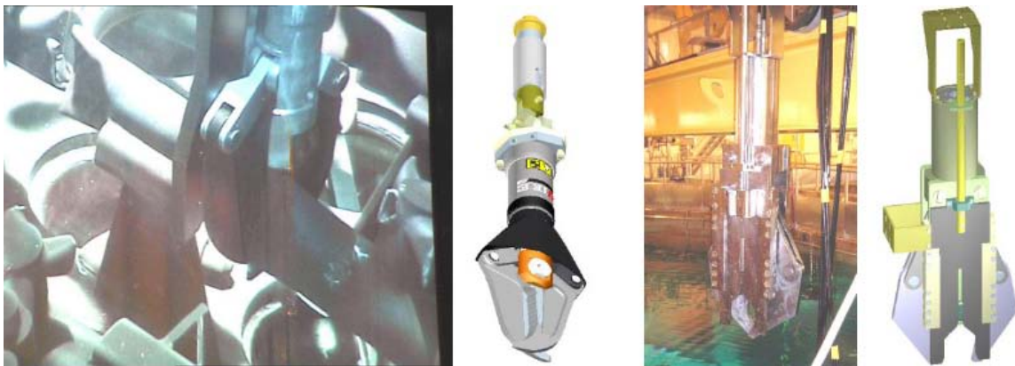
Figure A1-1. Shearing tools used to cut the core spray system and flat bars on the core grid.
