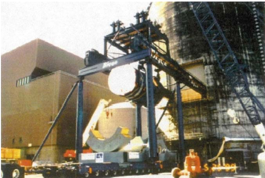
Figure A1-29. Removal of the Big Rock Point Pressure Vessel via a new side access.
