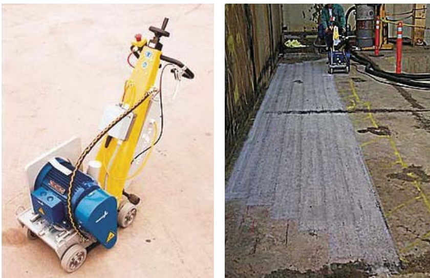
Figure A1-16. Marcris Floor Shaver and the resulting floor surface.
