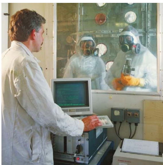
Figure 3-7. Manual dismantling operations utilizing Re-usable Modular Containment (RMC).
