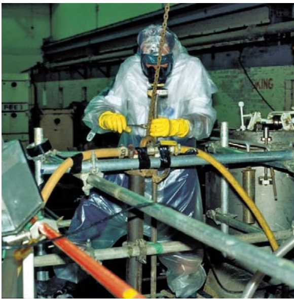
Figure 3-9. Preparation work prior to plant dismantling operations.
