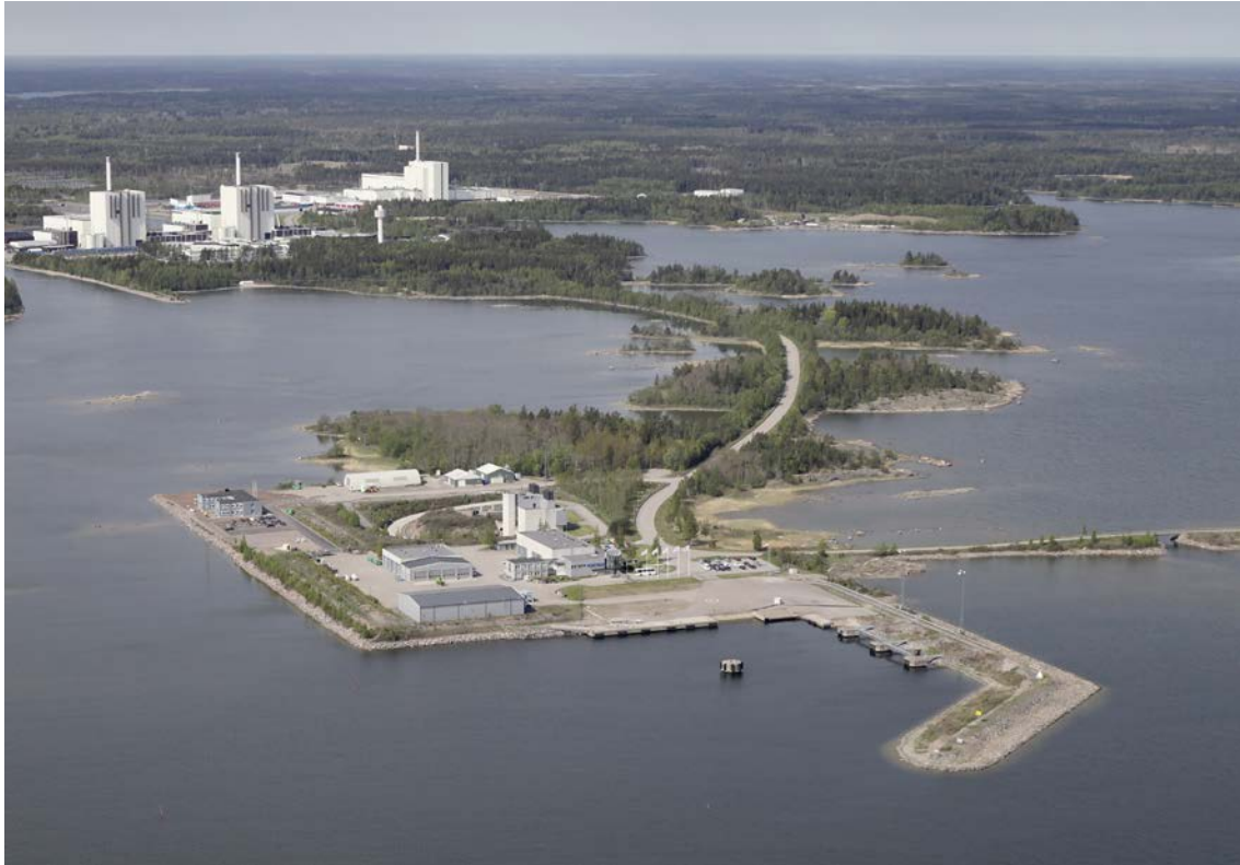
Figure 1-2. The surface part of the SFR facility in the Forsmark harbour with the Forsmark nuclear power plant in the background.
